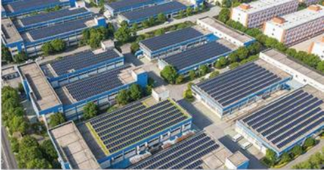
Industrial and Commercial Energy Storage Solutions ( User Side )
