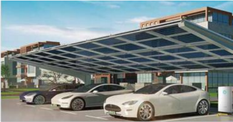
Integrated Solution of Solar Storage and Charging ( User Side )
